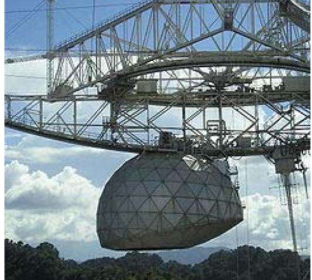
**Fig. 10.2. View of the beam steering mechanism. The wave length range of operation covers 3 cm – 1m.**
